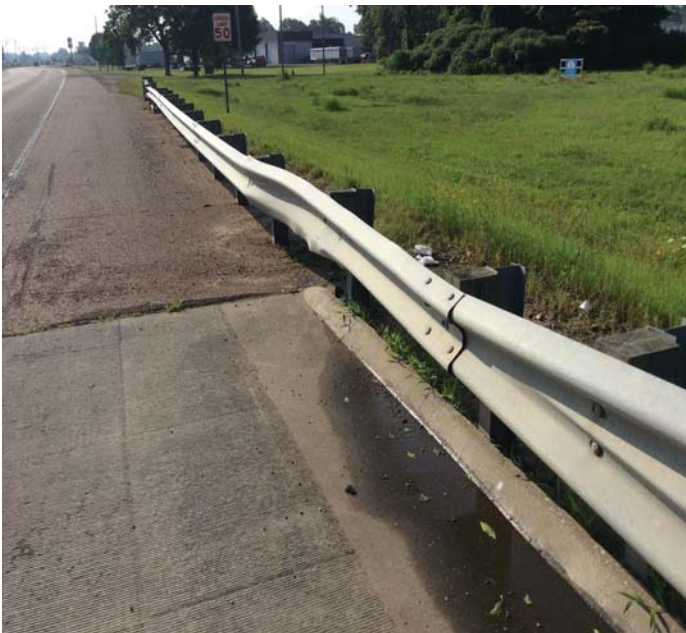
PHOTO 1 Description Abutment 2 right approach rail has collision damage 20' from bridge end.
