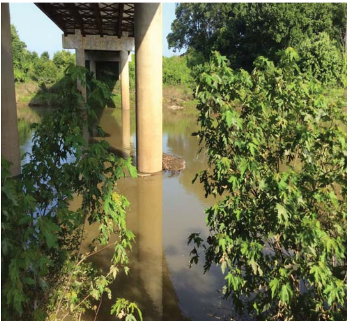
PHOTO 1 Description Small drift at bent 4 left side.
