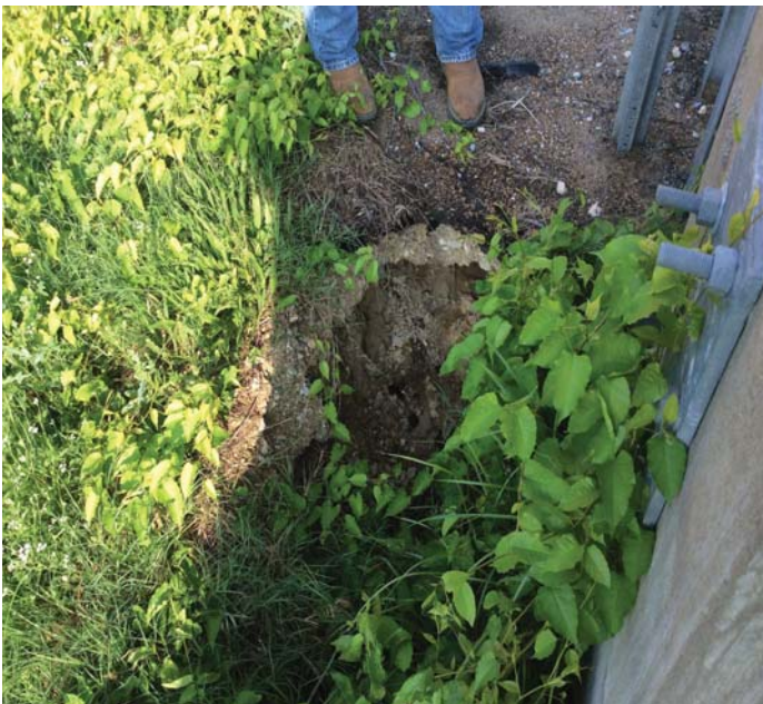
PHOTO 1 Description Abutment 1 right side at start of concrete bridge rail has 2' x 2' x2' deep erosion hole.
