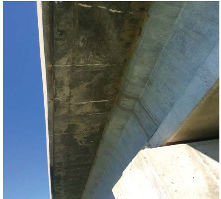
PHOTO 2 Description Overhang above bent 2: transverse cracks with efflorescence staining. Typical condition of the overhangs in the prestressed concrete girder units.
