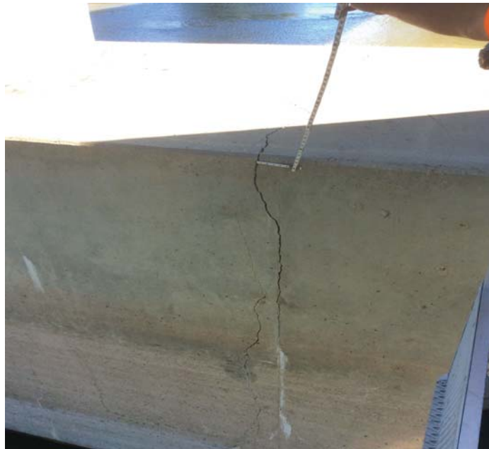
PHOTO 1 Description Pier 1 between column 2 & 3: large vertical crack (1/2" thick) in the sub cap. A crack similar between column 1 & 2.
