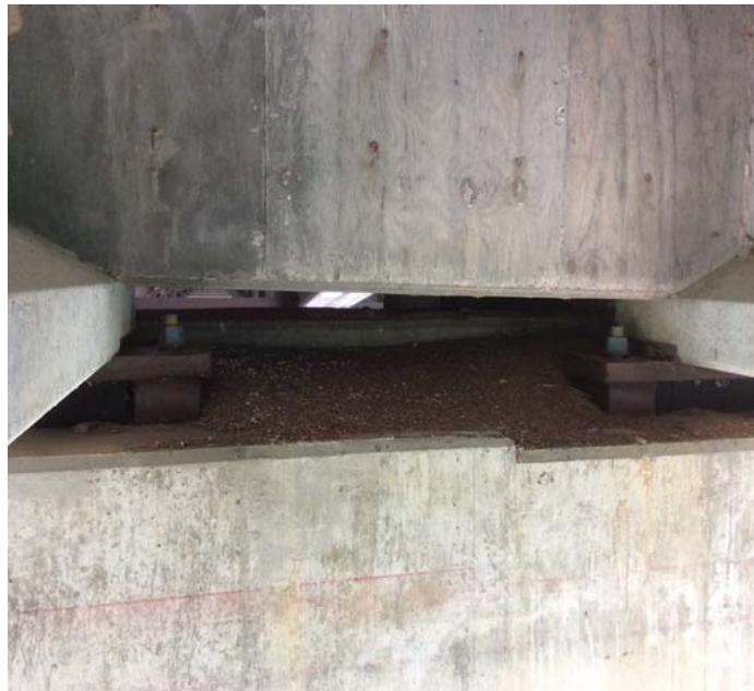
PHOTO 1 Description Bent 12: top of cap has a large amount of debris that has accumulated on it and around the bearings. This is the only joint on this bridge where this deficiency occurs.
