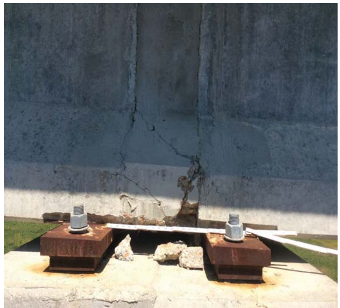
PHOTO 2 Description Bent 19 right side: spall and crack where prestressed girders are made continuous. Typical condition.
