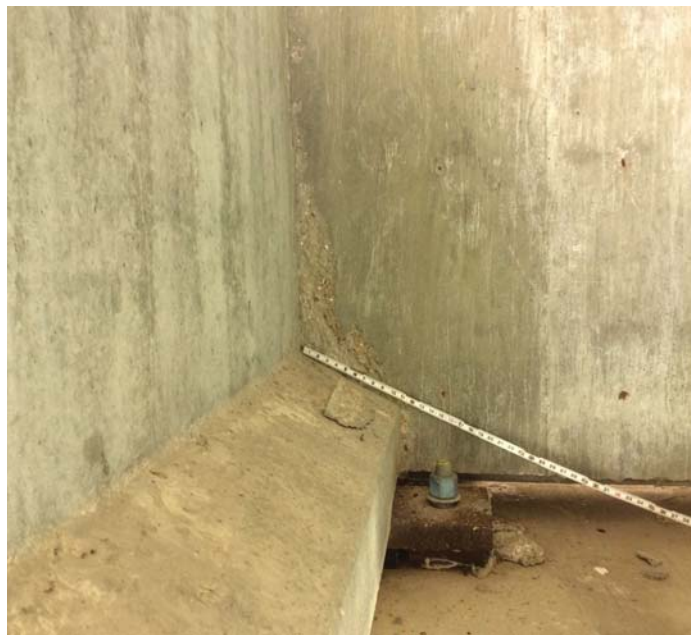
PHOTO 1 Description Span 9, backside of bent 10 where the prestressed units are made continuous, Spalls and delaminations are beginning to form around the girders. This is typical through out the bridge.
