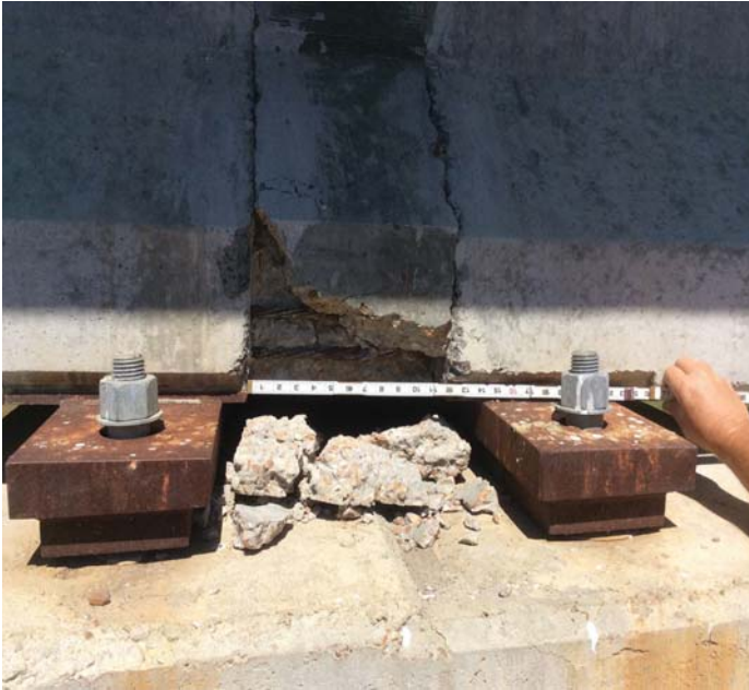
PHOTO 3 Description Rt. side bent 26: spall that is exposing reinforcing strands where the concrete girders are made continuous. Spalling and cracking in this area was typical throughout the prestressed units. This location was the worst case.
