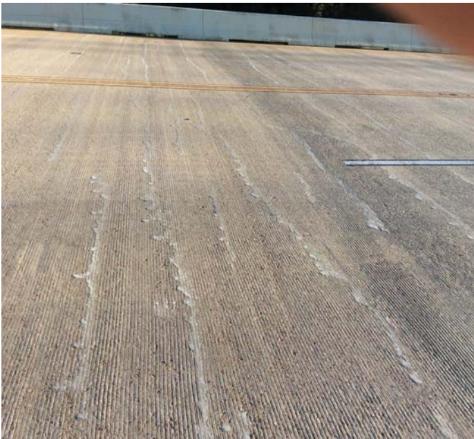
PHOTO 1 Description Span 3: the deck has numerous transverse cracks at 3 foot spacing that have been sealed in the past. Some of the seal is beginning to fail.
