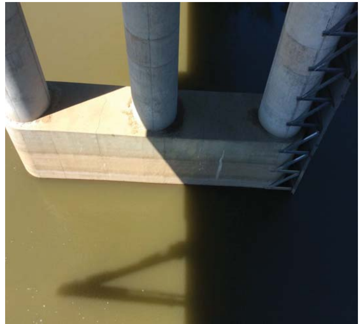
PHOTO 2 Description Back side Pier 1 sub cap: view looking from above at the large vertical cracks reflect through the pier.
