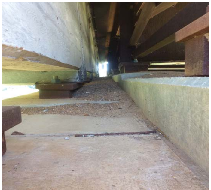
PHOTO 2 Description Bent 12 cap (side view): debris accumulating on top of cap and against the bearings.
