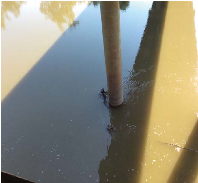
PHOTO 1 Description Bent 9 small drift.
