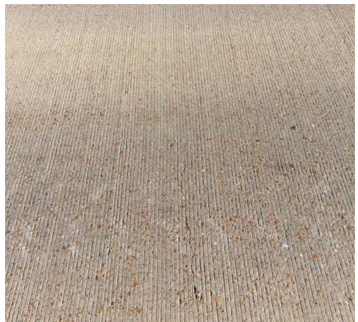
PHOTO 2 Description Typical deck cracks.
