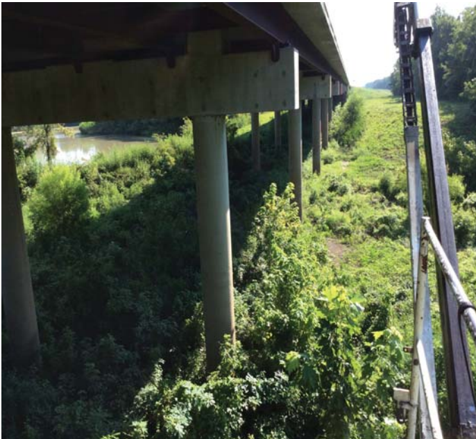
PHOTO 4 Description Small trees and vegetation growing under spans 11-26.
