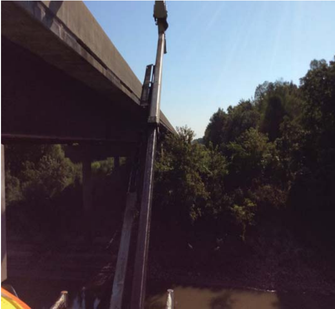
PHOTO 3 Description Tree growing beside bridge right side span 10 near bent 11.
