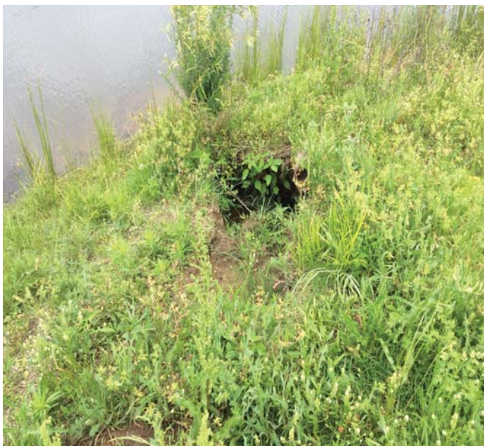
PHOTO 4 Description Hole in slope abutment #2 left side
