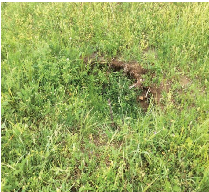
PHOTO 3 Description Hole in slope abutment #2 left side
