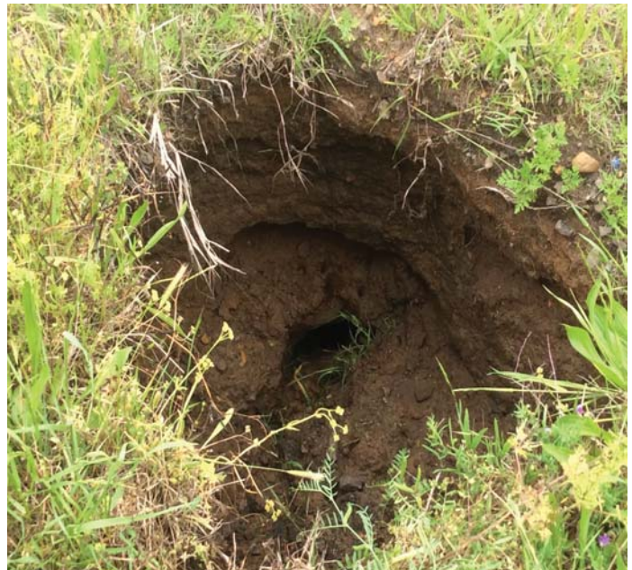
PHOTO 2 Description Erosion abutment #2 left side at drain
