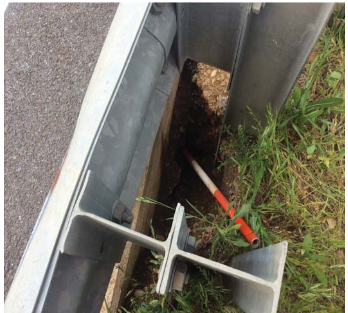
PHOTO 2 Description Hole eroded under approach curb abutment #2 left side
