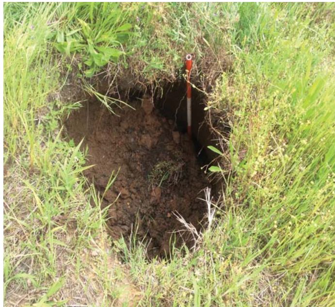
PHOTO 1 Description Erosion abutment #2 left side at drain
