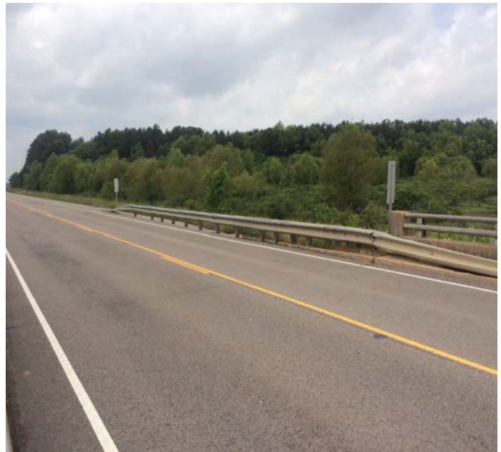
PHOTO 2 Description Abutment #1 left approach rail traffic damage
