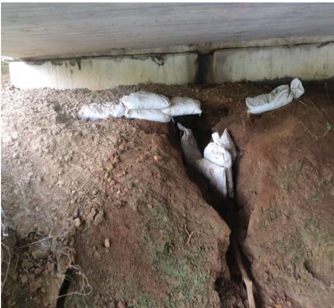
PHOTO 1 Description Erosion at abutment #2 left side.
