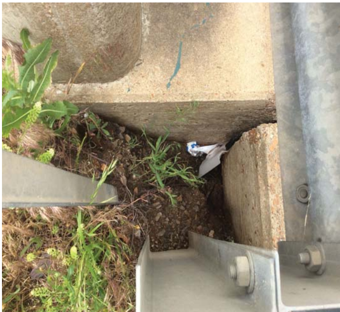
PHOTO 1 Description Erosion under approach gutter abutment #2 right side
