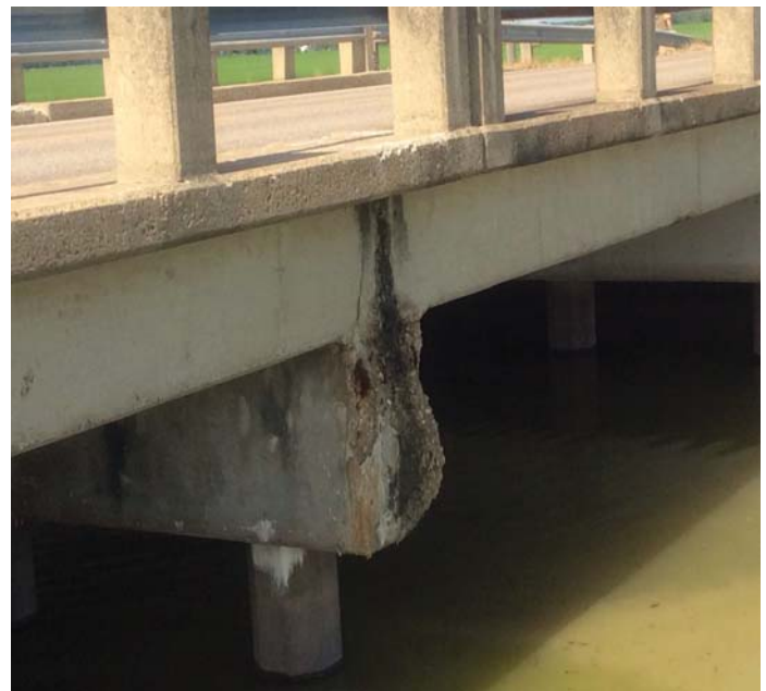
PHOTO 2 Description Bent #3 right end of cap and side of slab.
