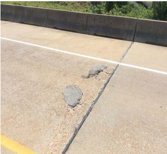
PHOTO 1 Description Spalls at bent 5.
