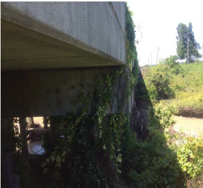
PHOTO 1 Description Vegetation growing onto bents.
