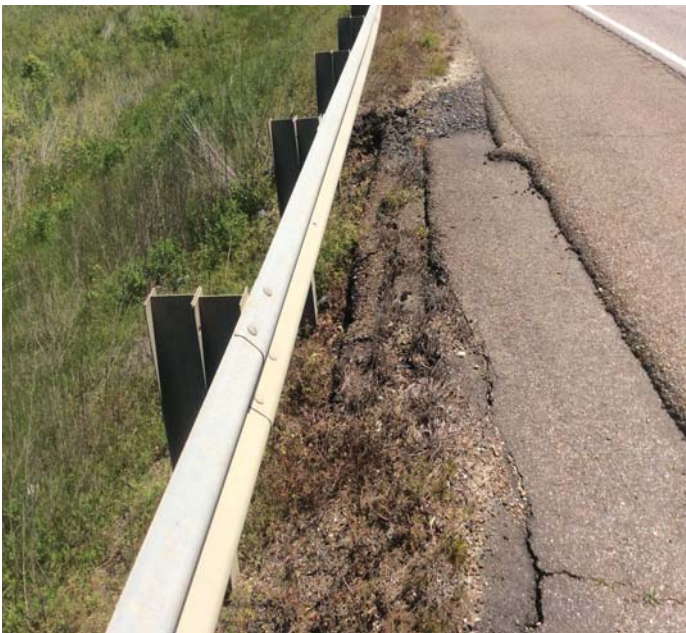
PHOTO 1 Description Abutment 2 left side 40' from bridge end approach shoulder and rail is being undermined for 20'.
