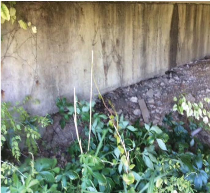
PHOTO 1 Description Abutment 2 cap undermined.
