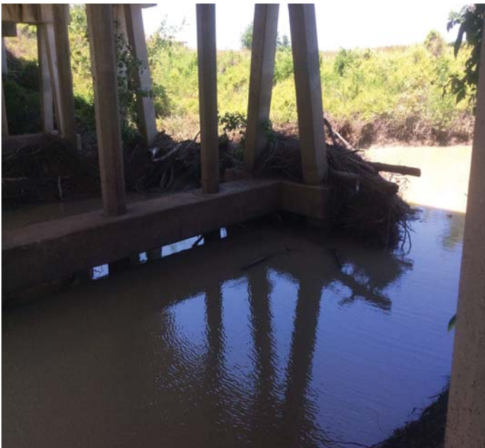
PHOTO 1 Description Drift left side of bridge.
