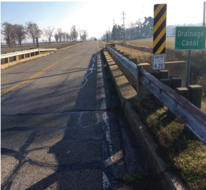
PHOTO 1 Description Vegetation is growing in gutters.
