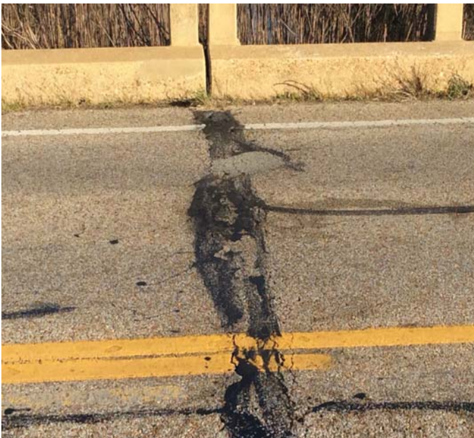
PHOTO 1 Description Span 1 pot hole repair.
