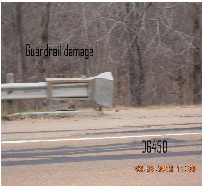
PHOTO 1 Description Terminal end post, collision damage.
