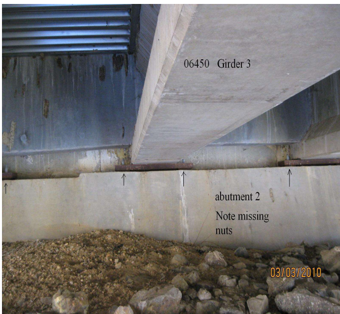
PHOTO 1 Description Abutment 2 girders 2, 3, and 4, anchor nuts missing.
