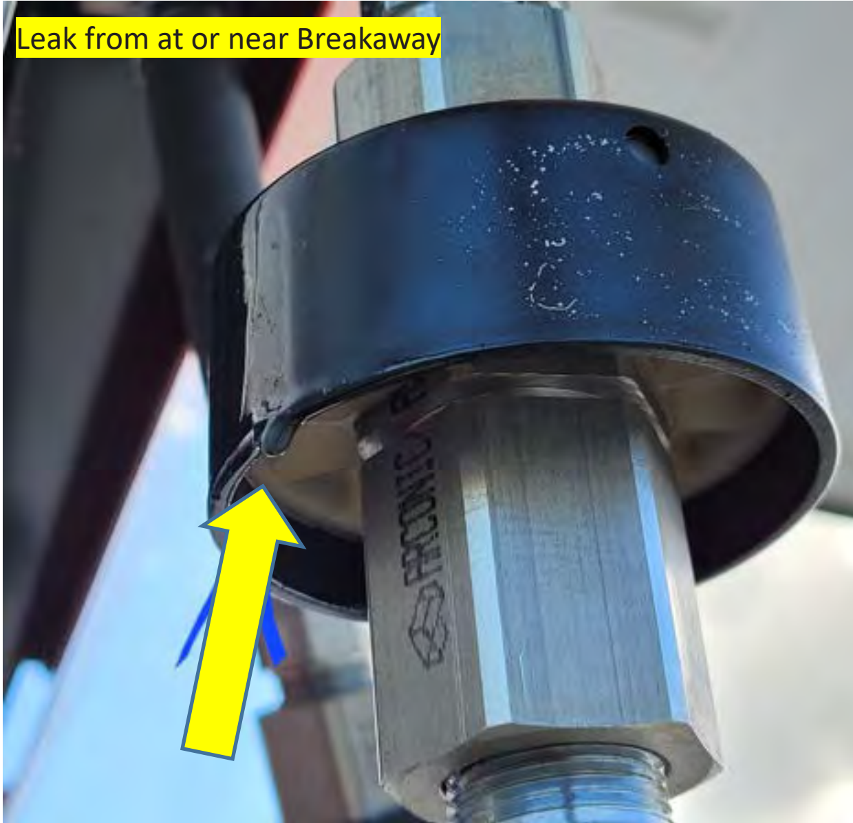
Leak from Nozzle, Swivel, or at thread
