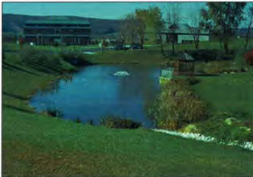
**Figure 1: Wet ponds can provide additional pollutant removal through settling**
