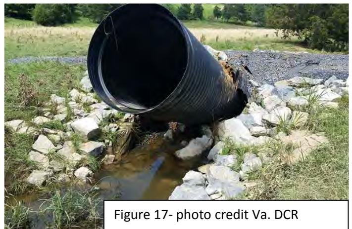
Figure 17: Poor placement of culvert resulted in buoyancy failure during high flow event. Culverts need 1 foot of cover and plastic pipes need to be weighted down.
