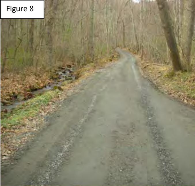
The inspections should assess the crown and roadway cross section; thickness and condition of the surface aggregate; and all drainage structures and flow paths.
