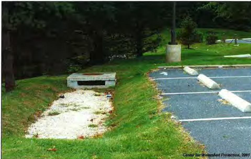
Figure 1: Infiltration Trench
