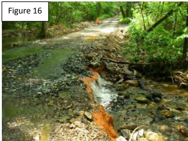
Figure 15: Inadequate culvert bedding combined with high flow depths causes piping; which is the loss of fill material. A headwall or riprap lining is needed.
