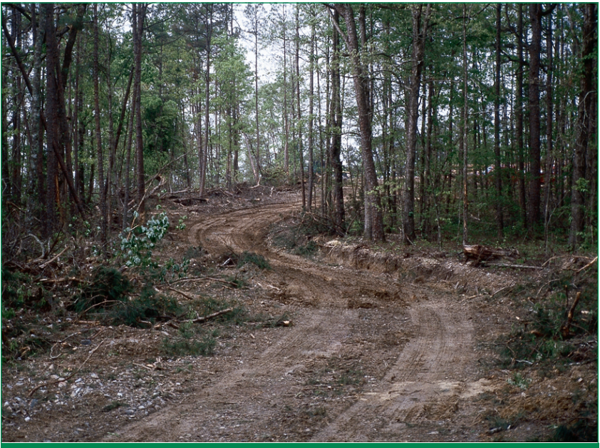
Temporary Active Road
