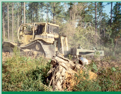
Mechanical Site Preparation
