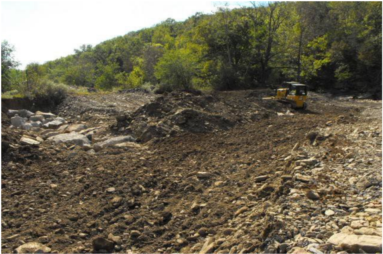
Upstream section: Bend-way # 8 and bank re-sloping.
