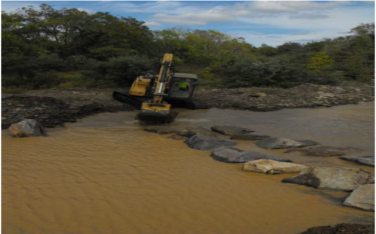
Bend-way weir # 5 installed.
