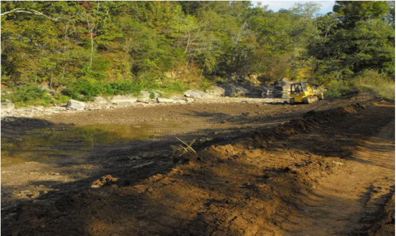
Downstream section banks being re-sloped.
