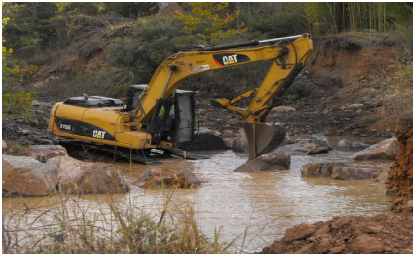
Bend-way weirs # 1, 2 and three installed, starting construction of bend-way weir # 4
