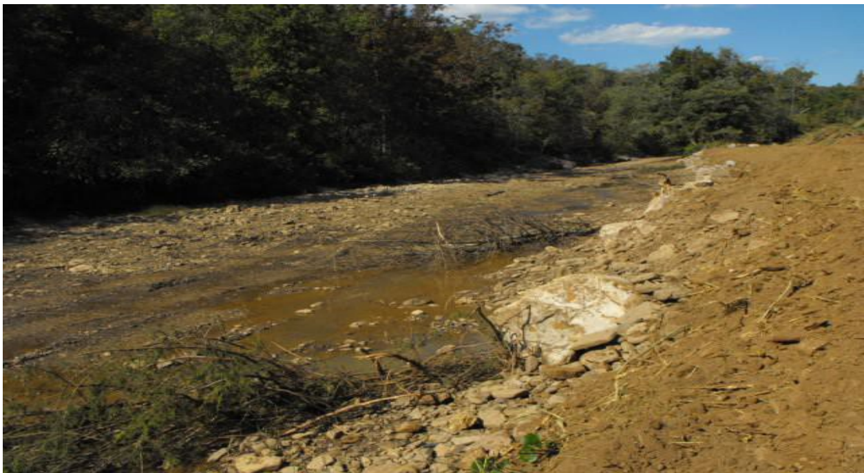
Downstream Section: Locked log and single stone Bend-way weirs installed.
