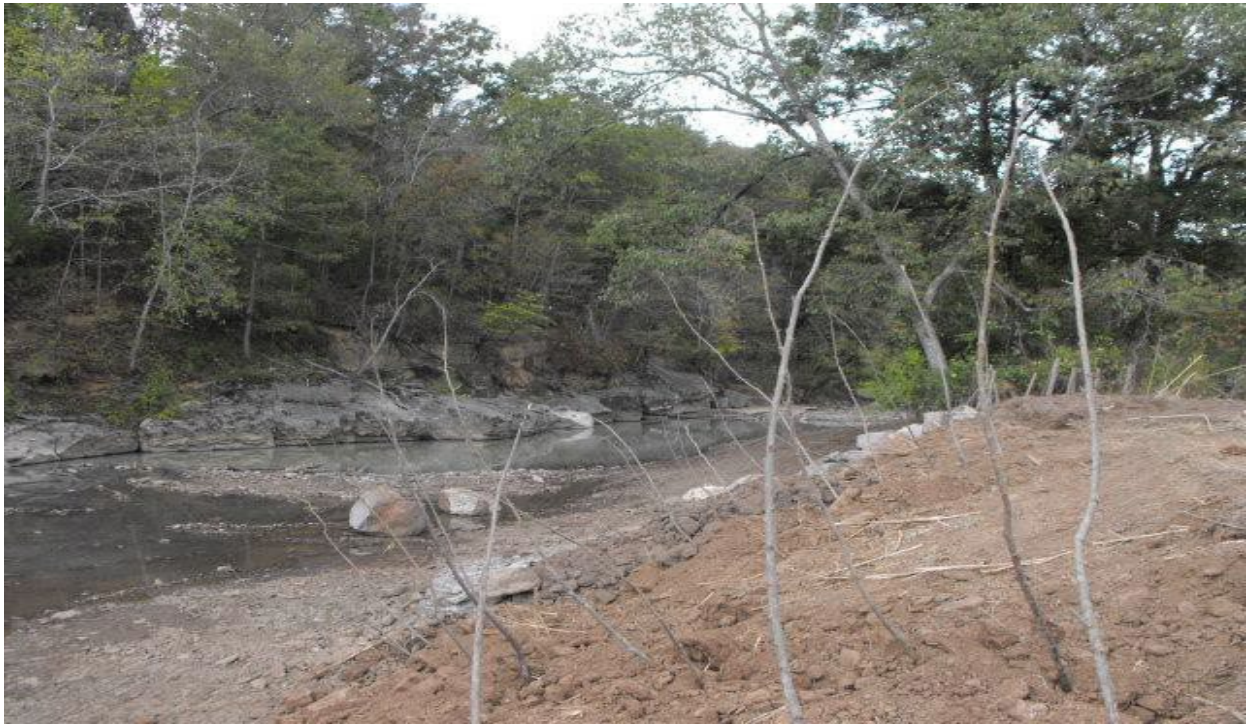
Downstream section: Willow and Sycamore poles in place (approximately 300).
