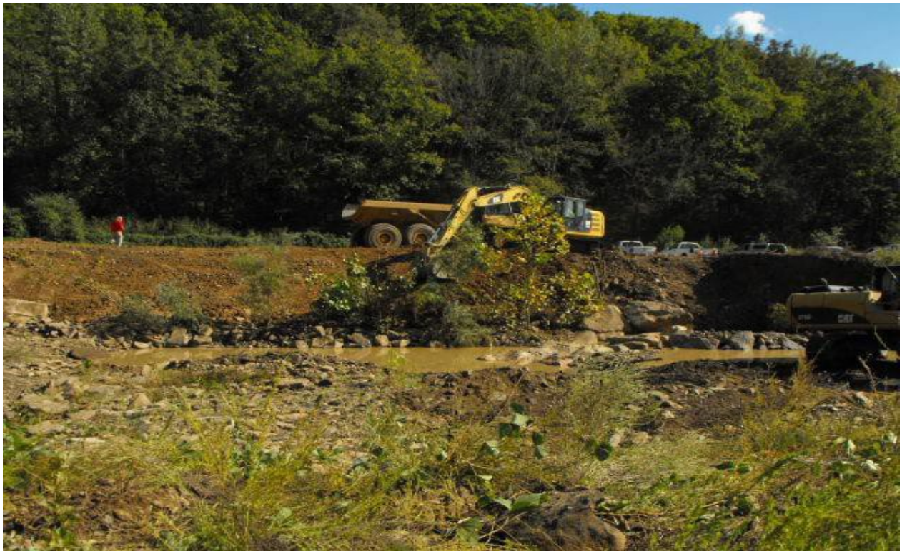
Upstream Section: LPSTP installed, transplanting vegetation to flood plain shelf.
