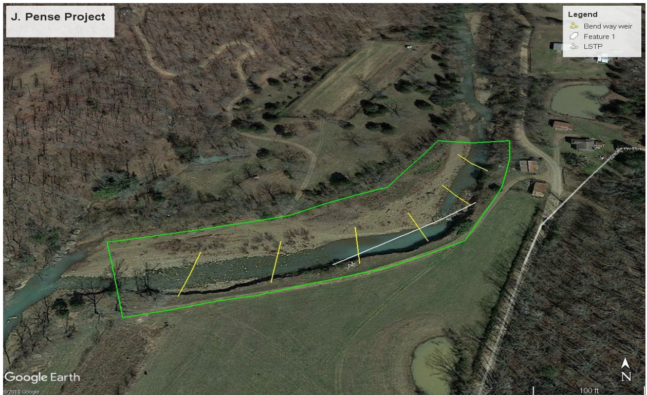
J. Pense project site.
