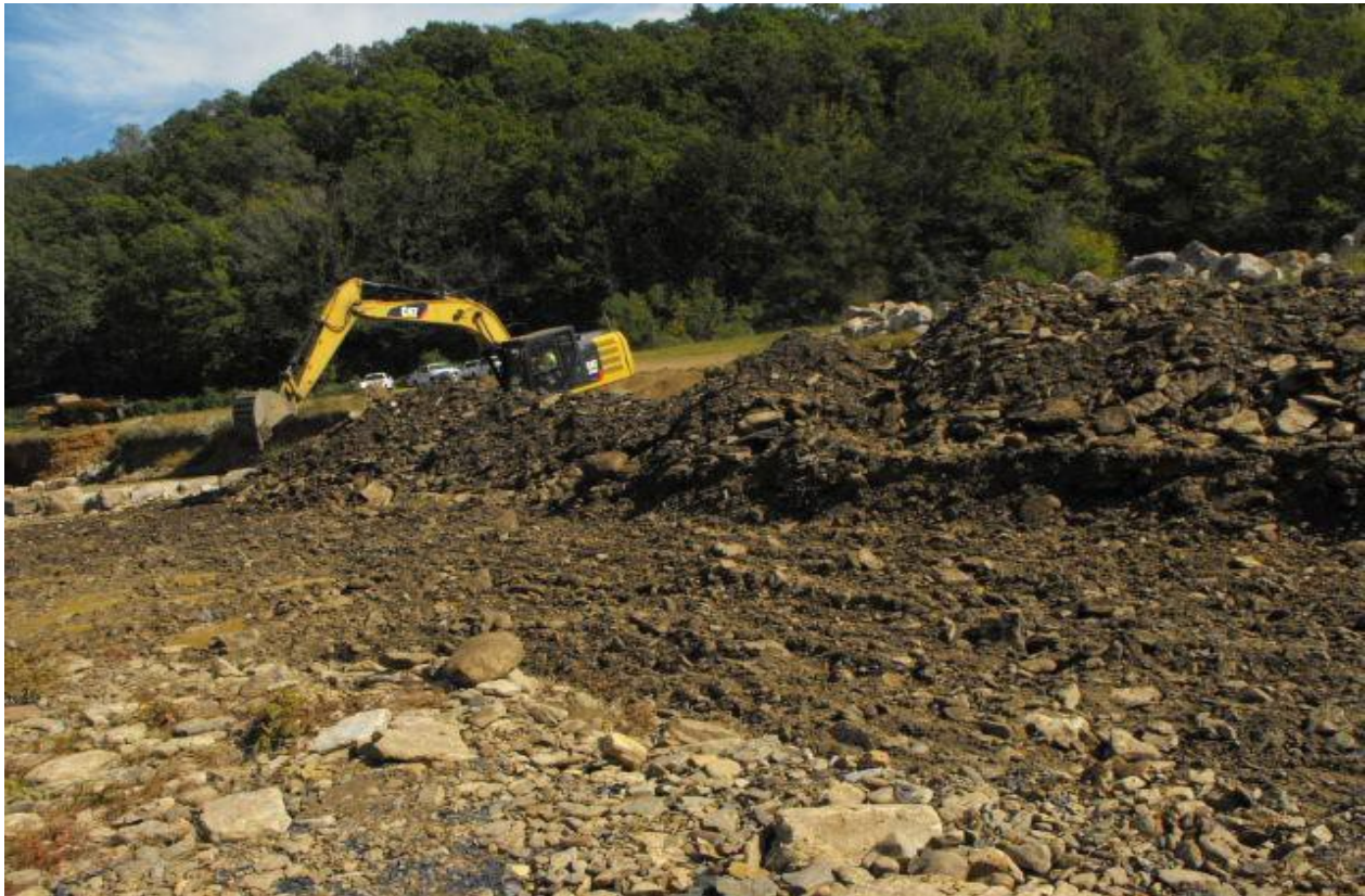
Upstream section: Stream bank being re-sloped.
