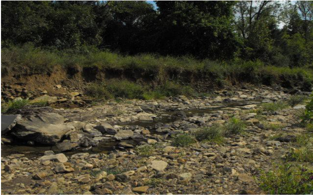
Downstream section prior to construction.
