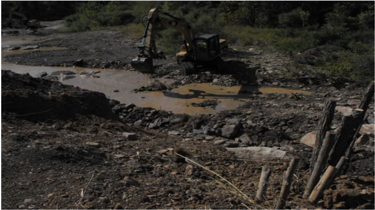
Upstream section: Longitudinal Peak Stone Toe Protection being installed.
