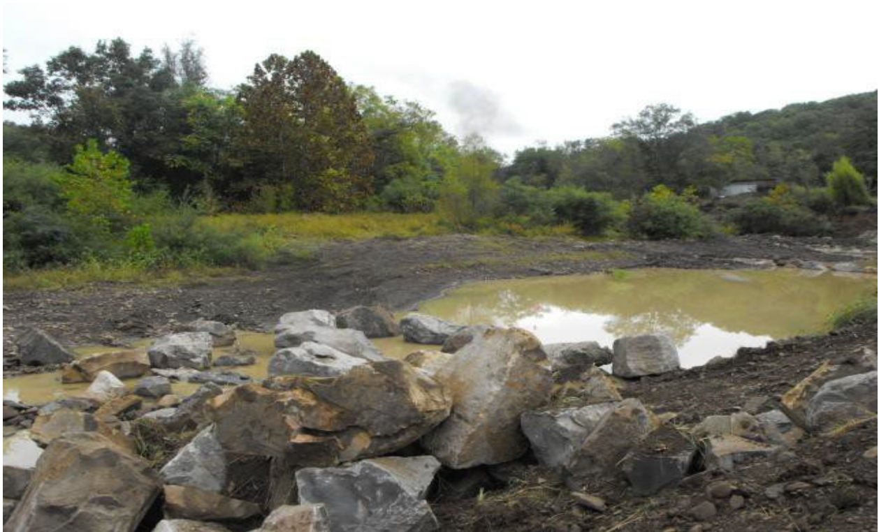
Road crossing and Bend-way weir # 6 being constructed.
