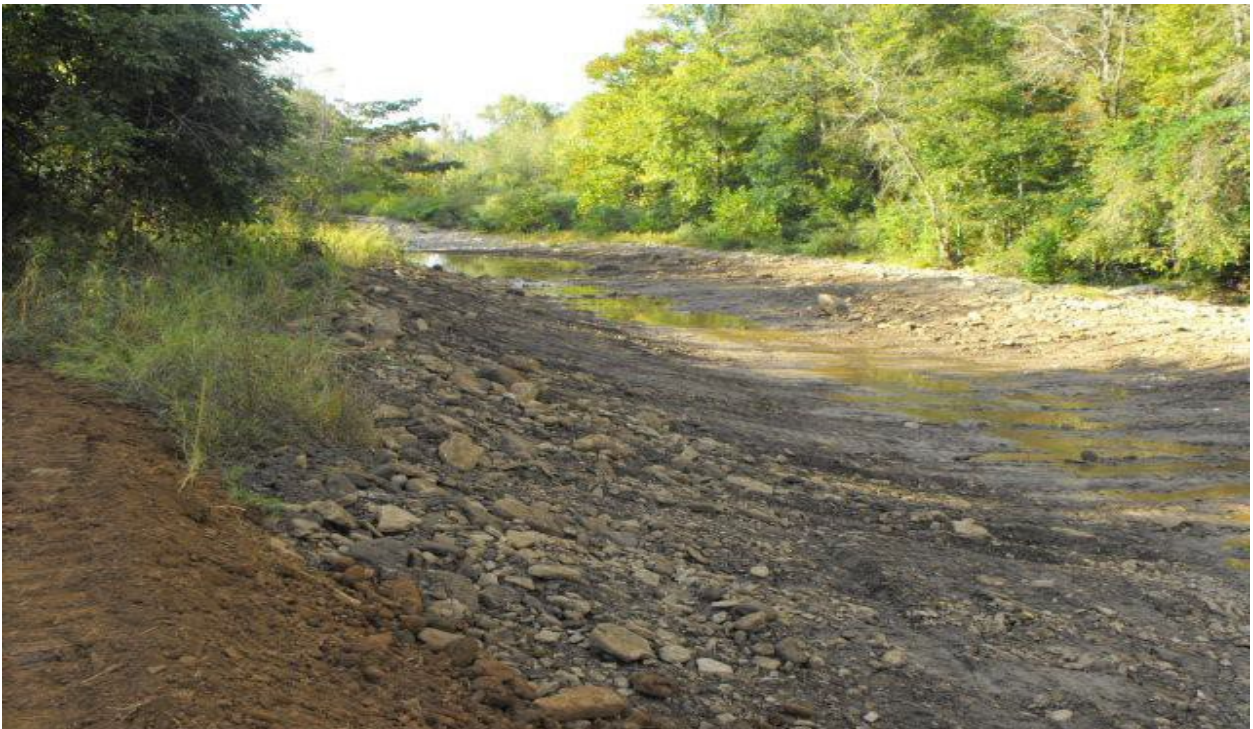
Downstream section banks re-sloped.
