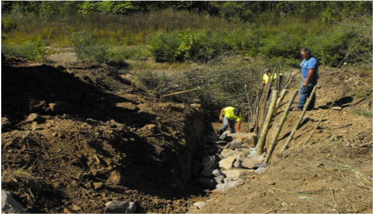
Key-lock # 1 with poles and stone added.
