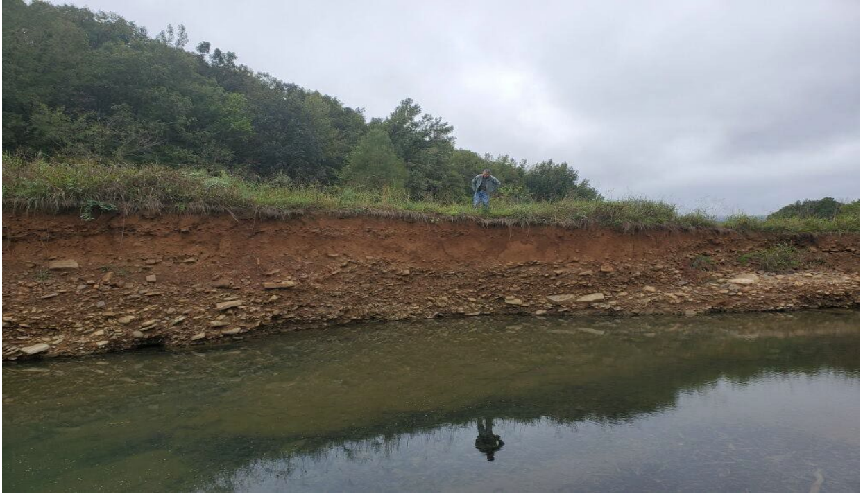
Upstream section prior to construction #1
