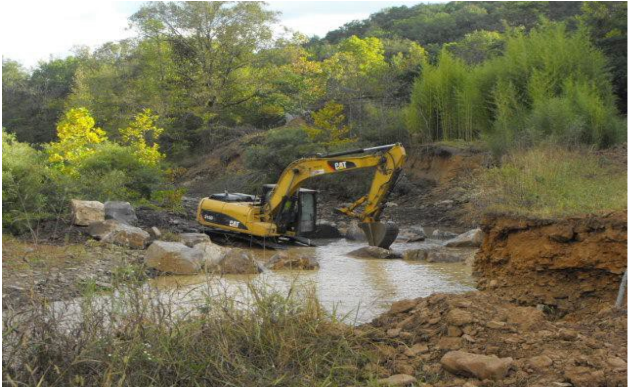
Bend-way weir construction.
