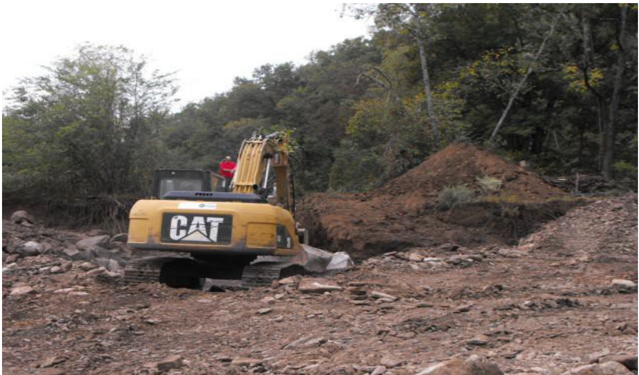
Key-lock and bend-way weir # 8 being constructed.
