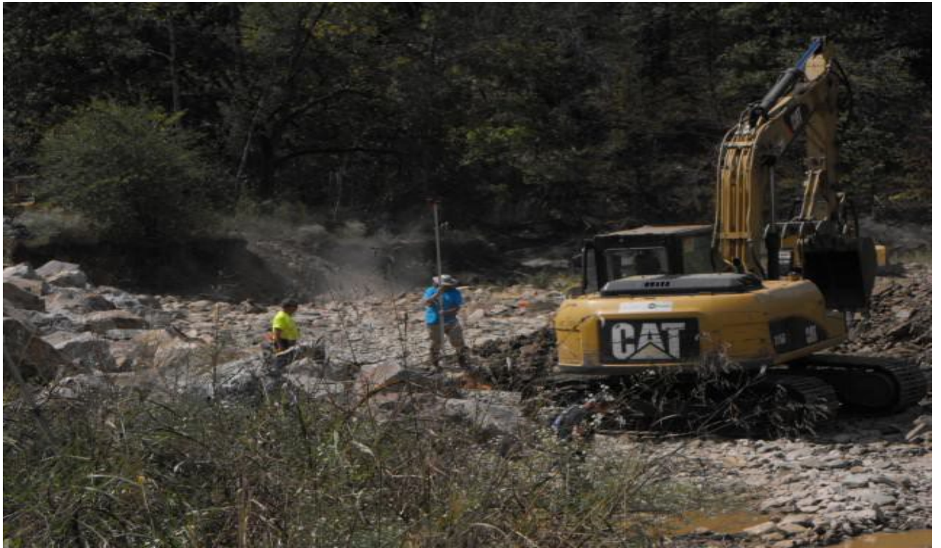
Bend-way weir # 7 sited for elevation drop.
