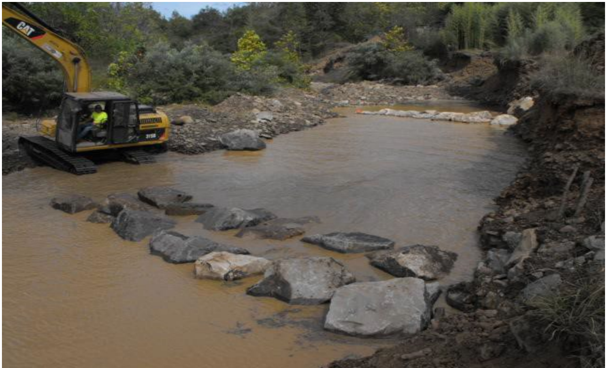
# 4 Bend-way weir installation.
